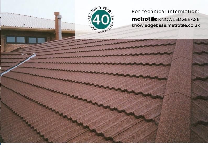
Whether you're a construction company or a homeowner, Metrotile is the consistent roofing supplier of choice for low pitch roof tiles. Our lightweight roofing can be installed at a pitch as low as 10 degrees which means it's often specified for flat to pitch roofing conversions, and has been successfully installed on homes to blocks of flats.
