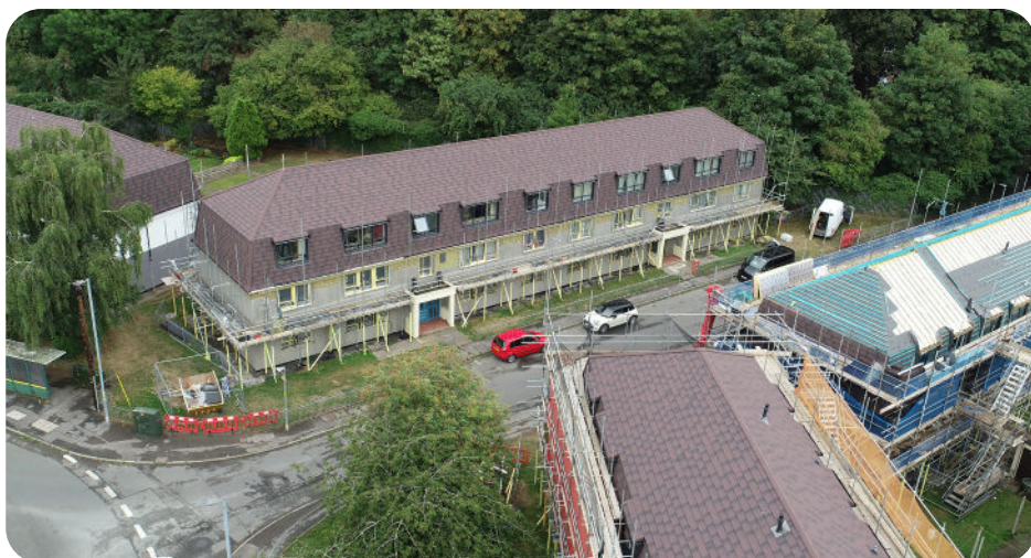
Above: 3 of the 7 completed blocks of successfully re-roofed Cornish Units in Metrotile's Burnt Umber Shingle Tile.
