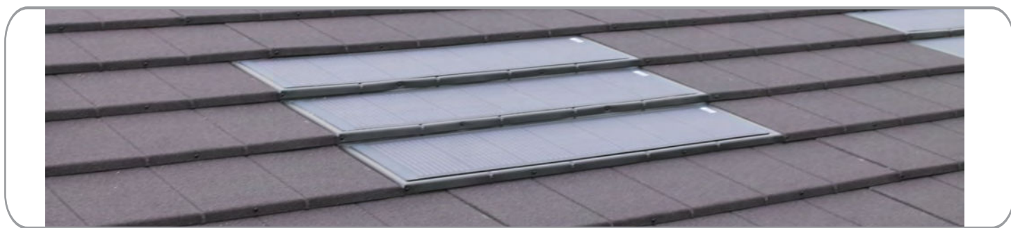
Metrotile uses Verditek 3x7 photovoltaic panels
