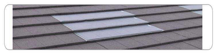
Metrotile uses Verditek 3x7 photovoltaic panels
